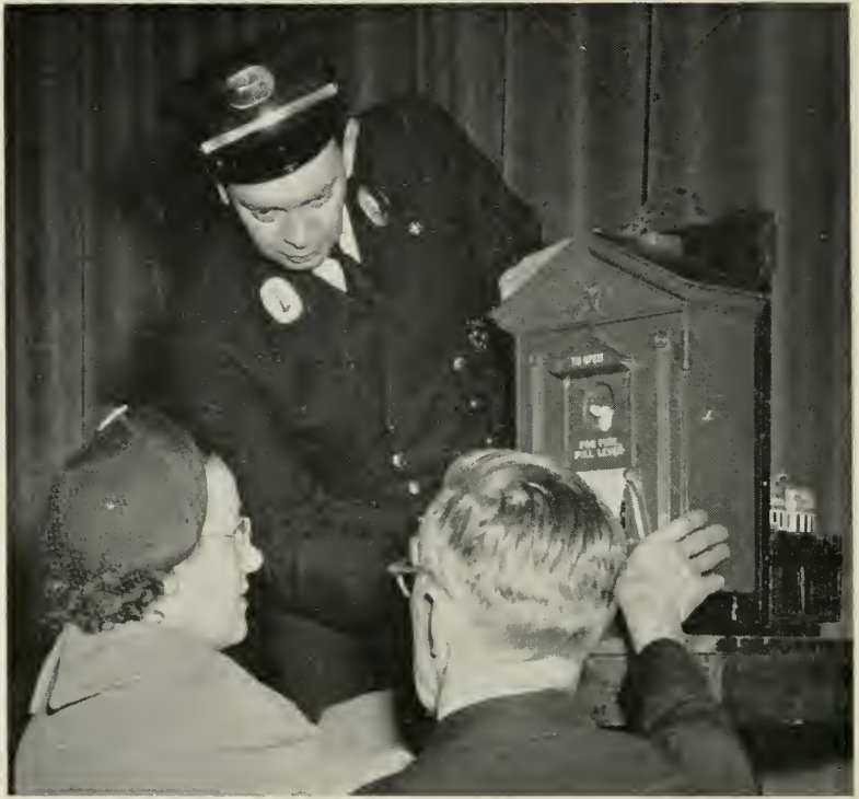
Fire Alarm Demonstration
